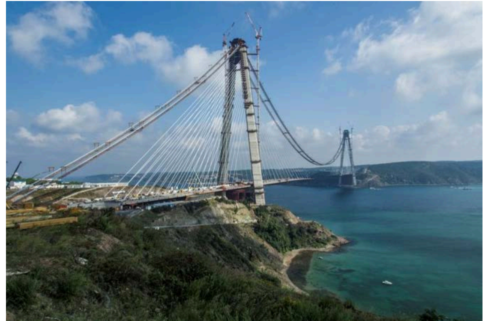
Textile reinforcement for the new Bosphorus bridge by solidian (c) 2017 solidian
